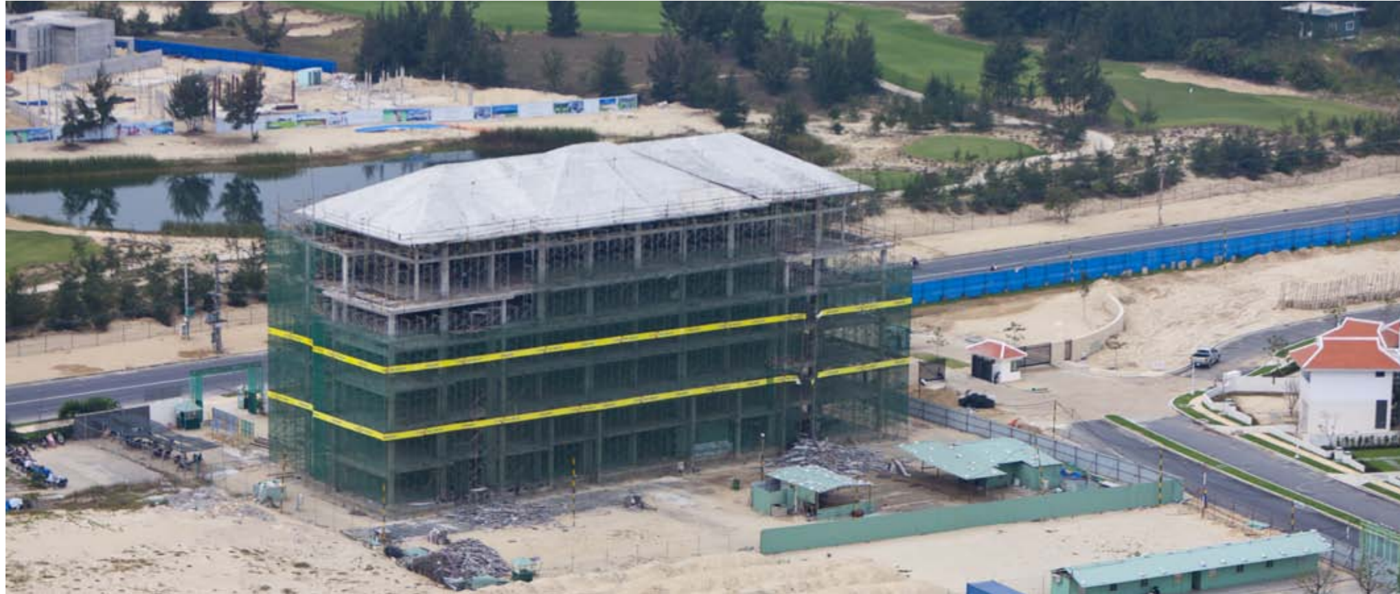
Construction of tower A is now well advanced at The Cham Condominium.
