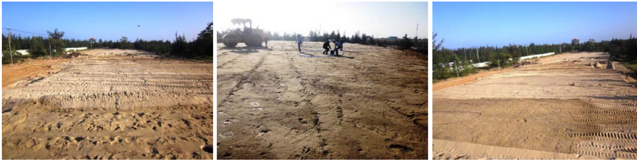
The Point site is cleared and ready for construction to start
